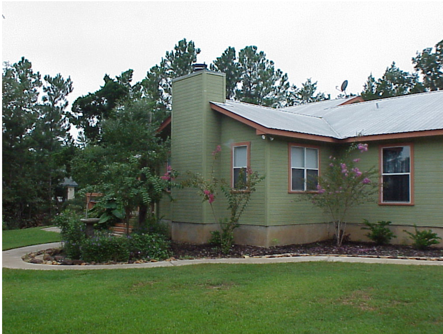
Excellent Defensible Space with Sidewalk Acting as a Firebreak
